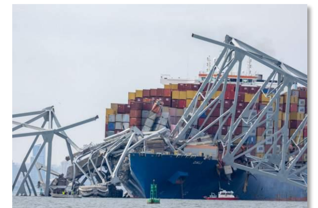
Collapse of Baltimore's Francis Scott Key Bridge after it was hit by the DALI. March 26 th 2024 Credit: Dwayne Senior/Bloomberg
